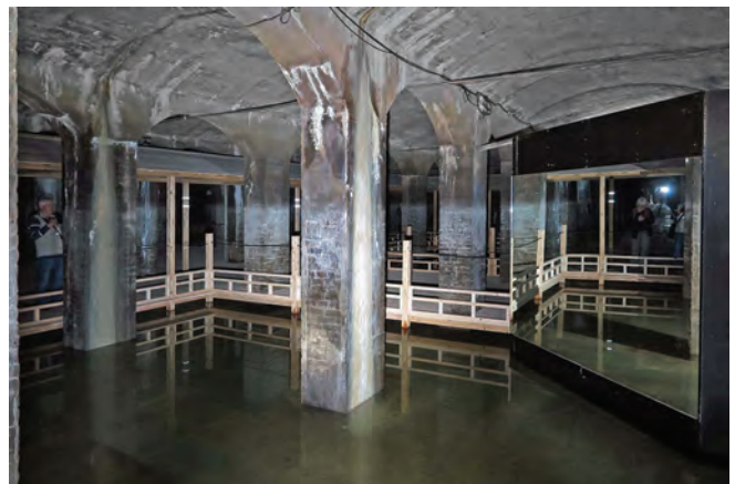
The interior of the Cistern. The walkway forms part of the art installation as shallow water now completely covers the floor of the reservoir. The masonry pillars and cast concrete roof can also be seen
